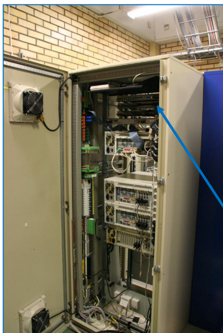
Cabinet before we started
